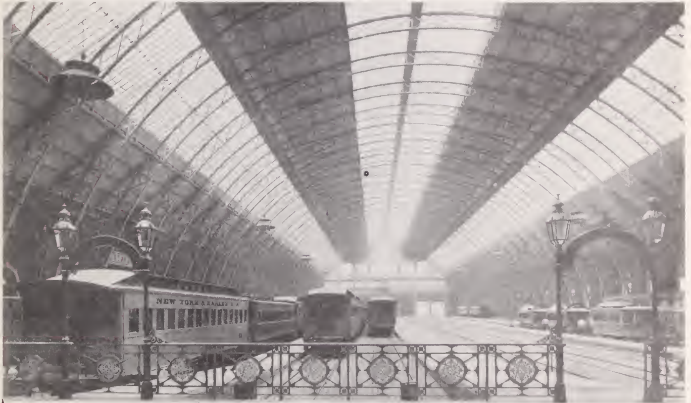
Fig. 5. Train shed, Grand Central Depot, R.G. Hatfield, engineer. This 1873 view shows the arch-ribbed shed shortly after opening. Note the horse-drawn cars at the right and the glass-and-metal curtain wall at the northern end.
